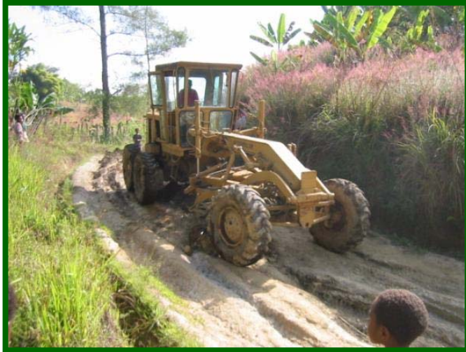
Rehabilitation with Equipment by Contractor
